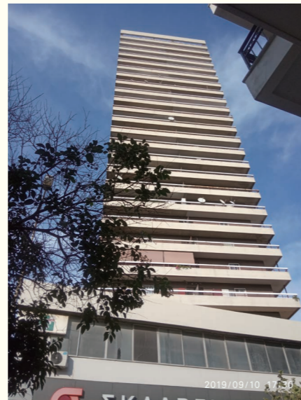
'Apollo Tower residential high-rise building side view' by Peloponnisios available at https://commons.wikimedia.org/wiki/File:Apollo_Tower_residential_high-rise_building_side-view.jpg under the Creative Commons Attribution-Share Alike 4.0.
